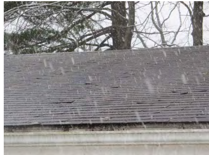
Roof shingles exhibit signs of age-related wear
