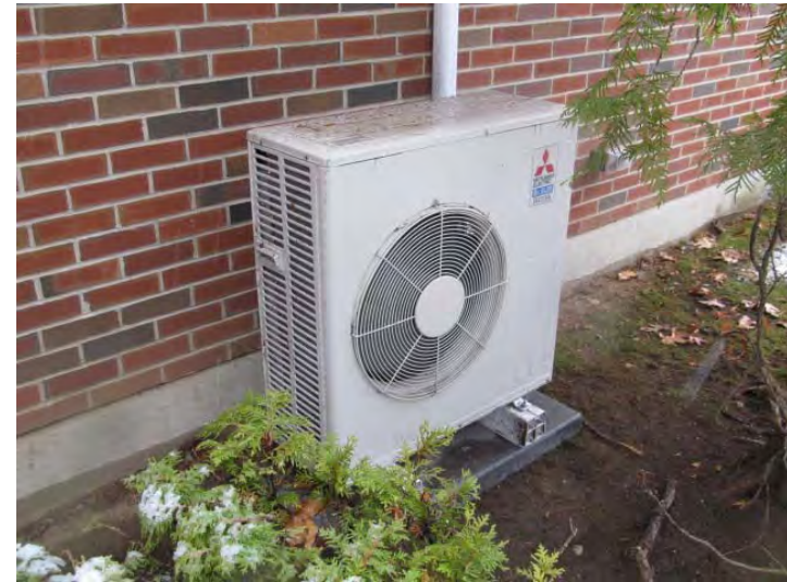
Recently installed exterior condenser unit for heat pump serving interior spaces at Community Building
