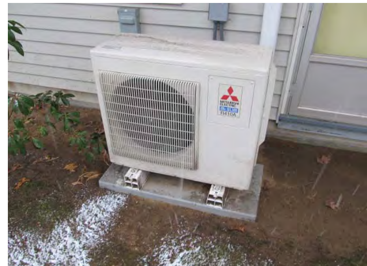
Typical, exterior-mounted, condenser for recently installed heat pumps that serve unit heating/cooling needs
