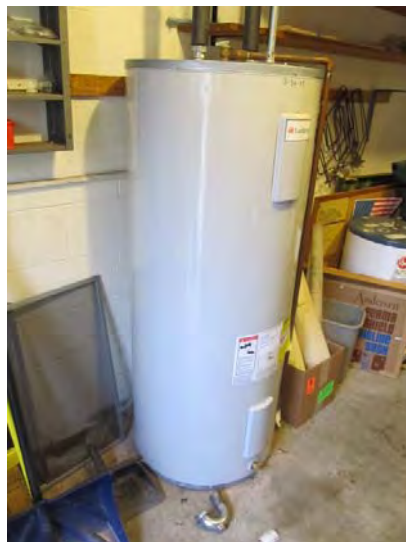
Electric domestic hot water tank serving spaces within Community Building
