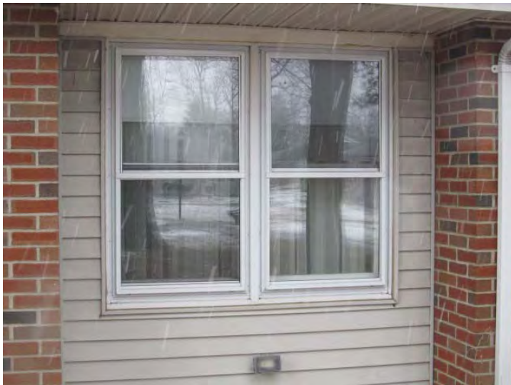
Original wood sash windows and newer aluminum-framed exterior storm windows are typical
